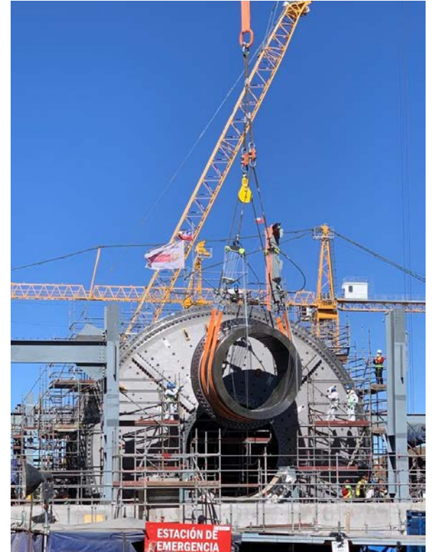
SAG #1 trunnion installation, August 2020
